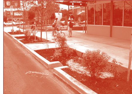
Example of on-street bioretention areas— Portland, Oregon.
